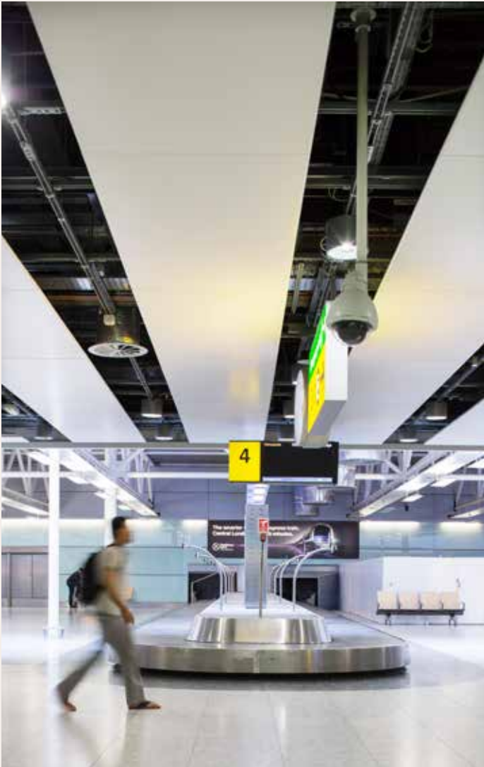
Heathrow T3, Immigration and Baggage Hall Refurbishment
