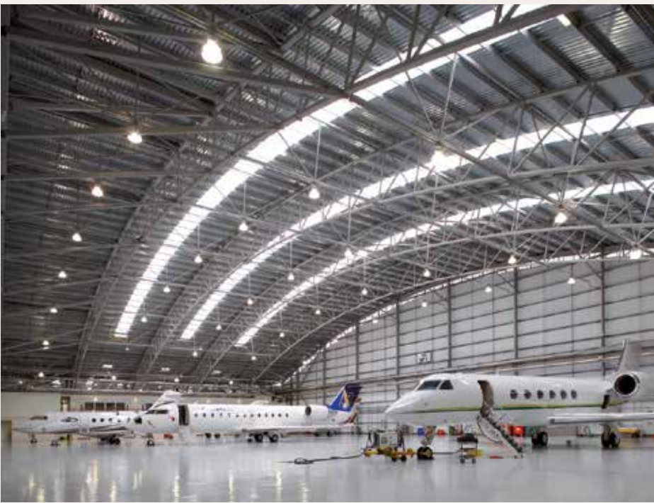
The maintenance and hangar facilities are column free, utilising an innovative design created in tandem with the structural engineers, Buro Happold.
