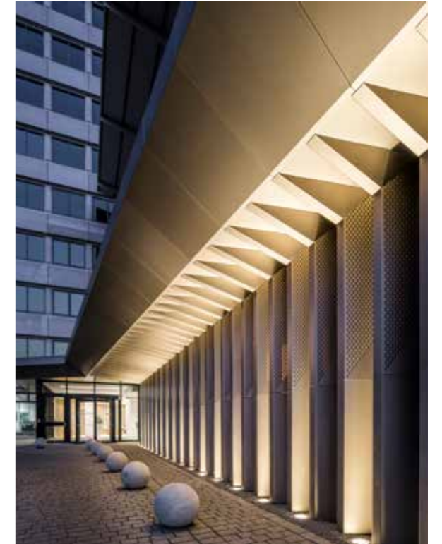
The Switch entrance.
