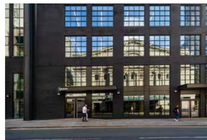
Quay Street facade.
