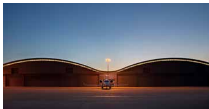
Industry & Technology / Farnborough Airport Hangars.
