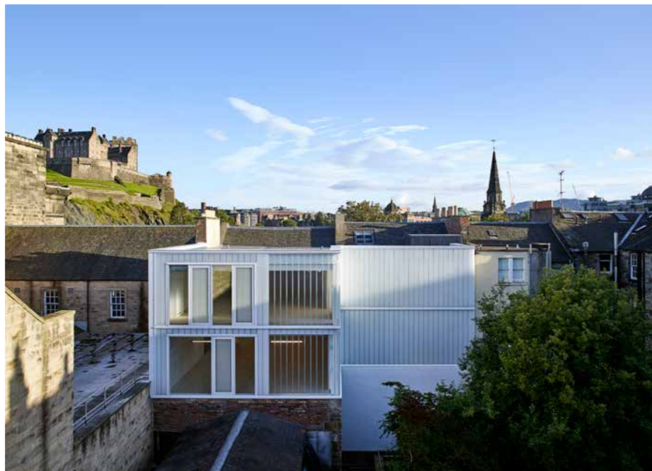
Contemporary extension to the rear of the building.
