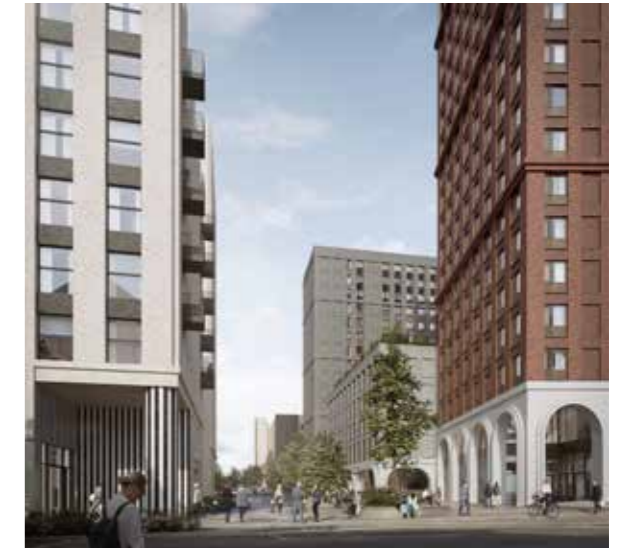
Plot A and B looking west.
