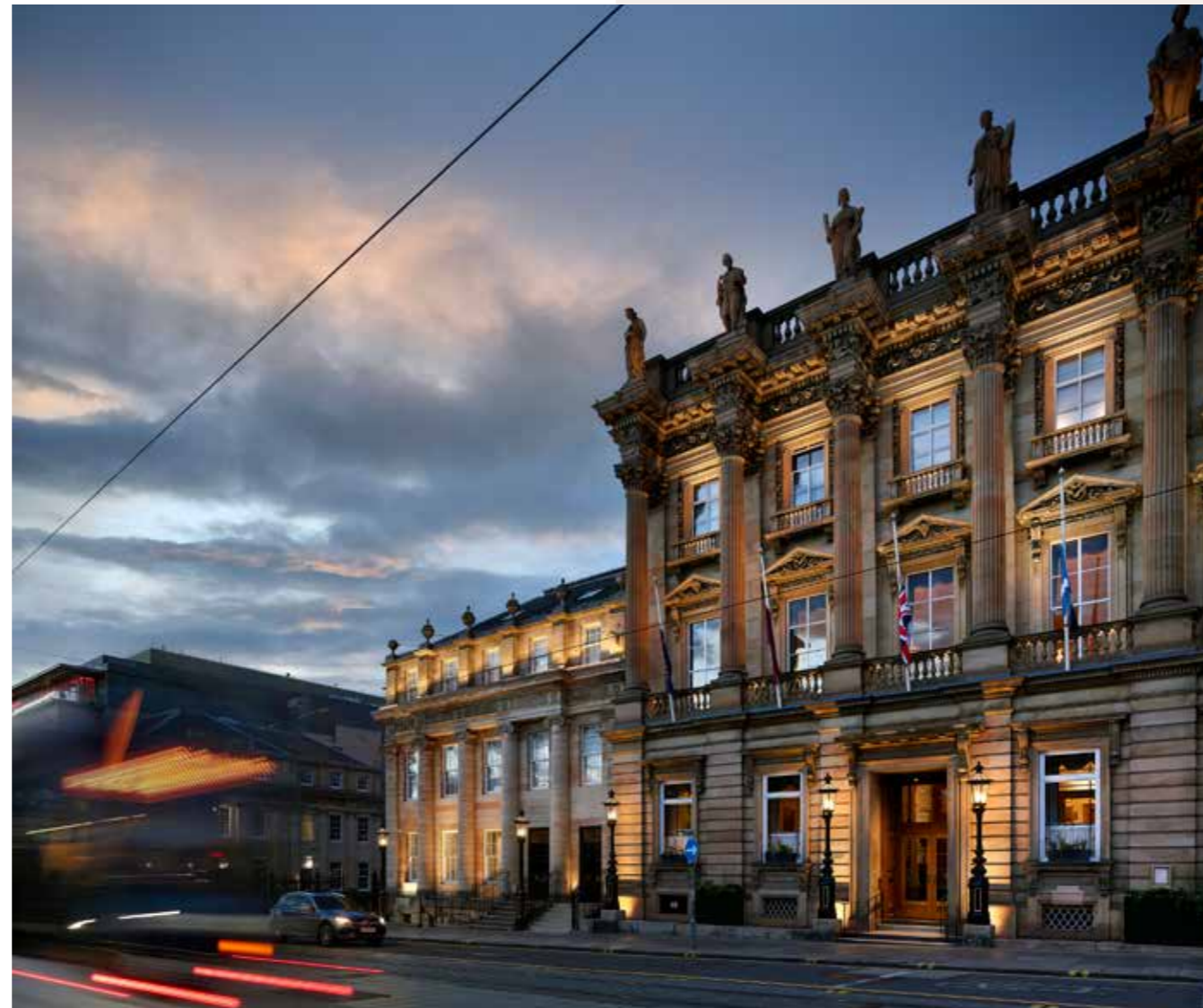
No. 39 St Andrew Square entrance.
