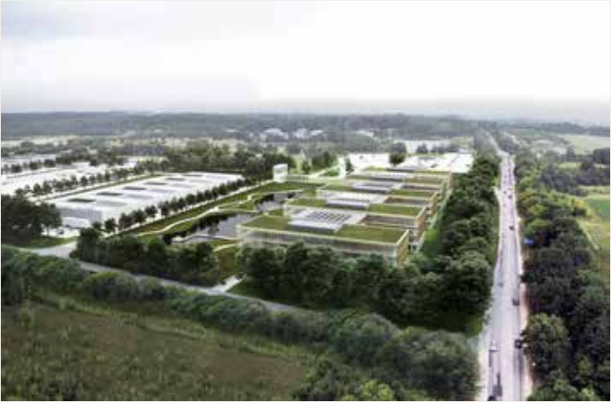
Proposed aerial view from North West
