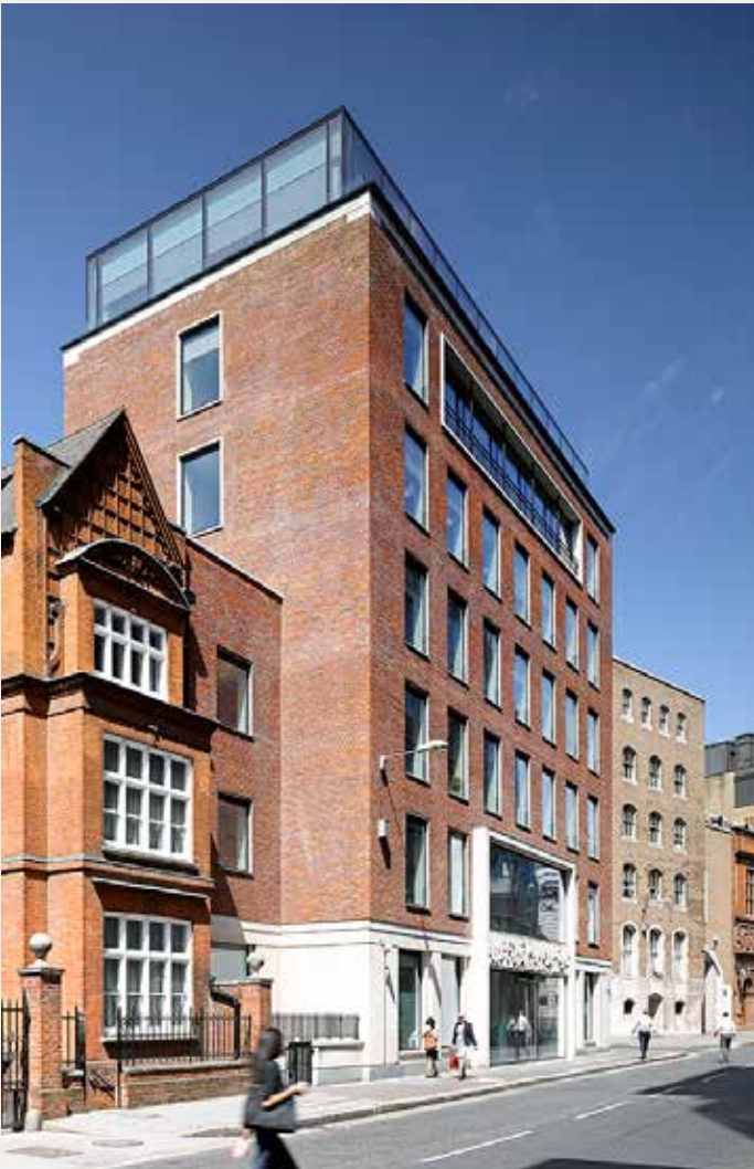
St Paul’s House entrance on Warwick Lane.
