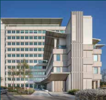
The Switch Slough
