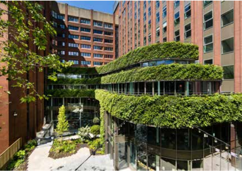
View from the courtyard.
