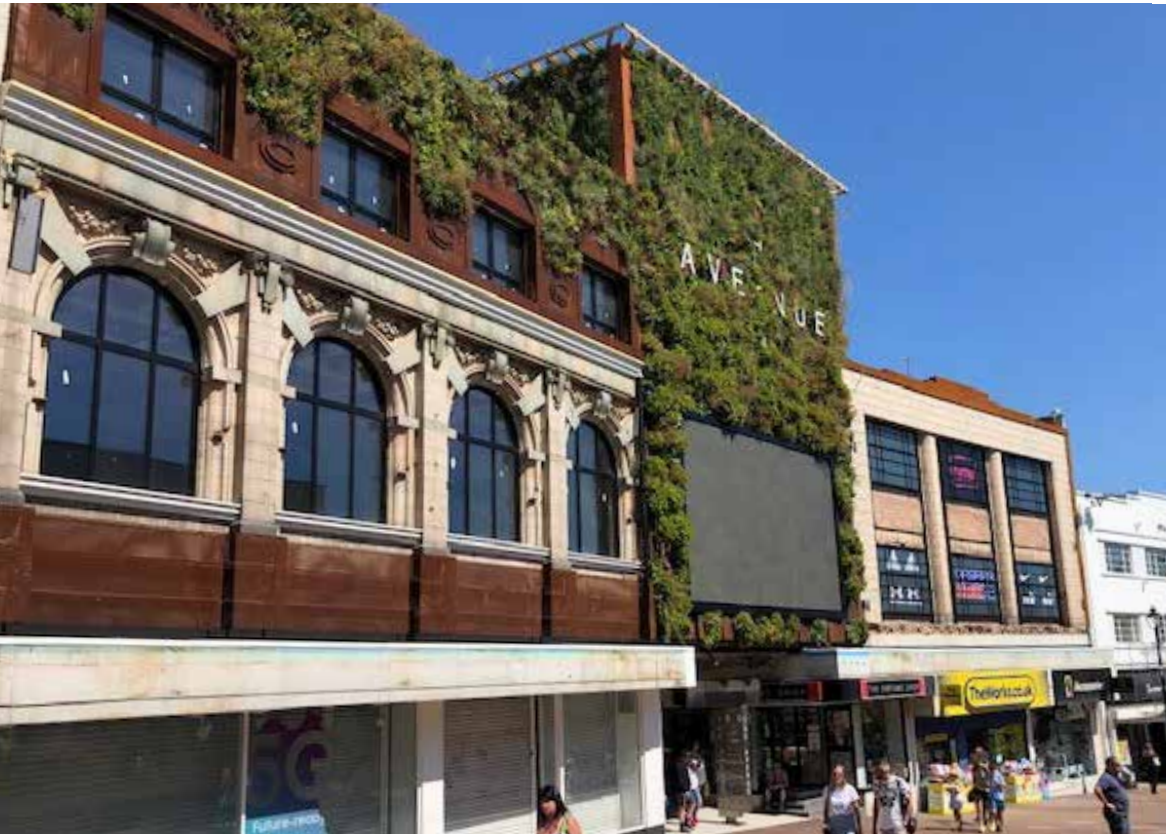
Commercial Road facade.
