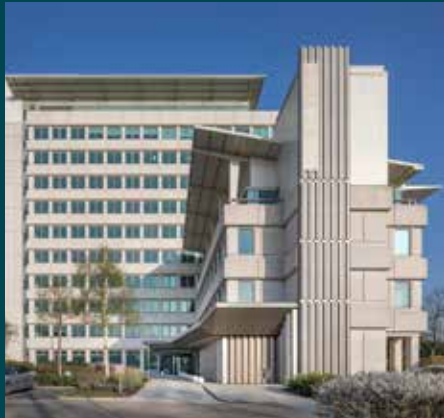
The Switch Slough
