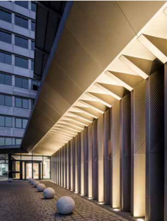
The Switch entrance.
