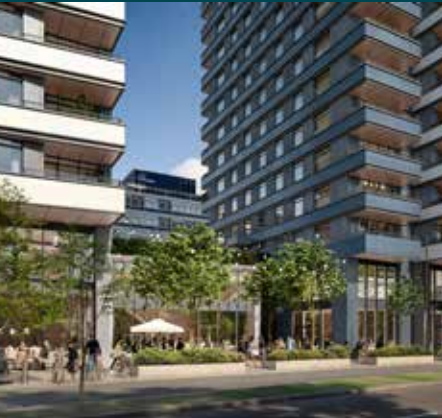
Tolworth Tower London
