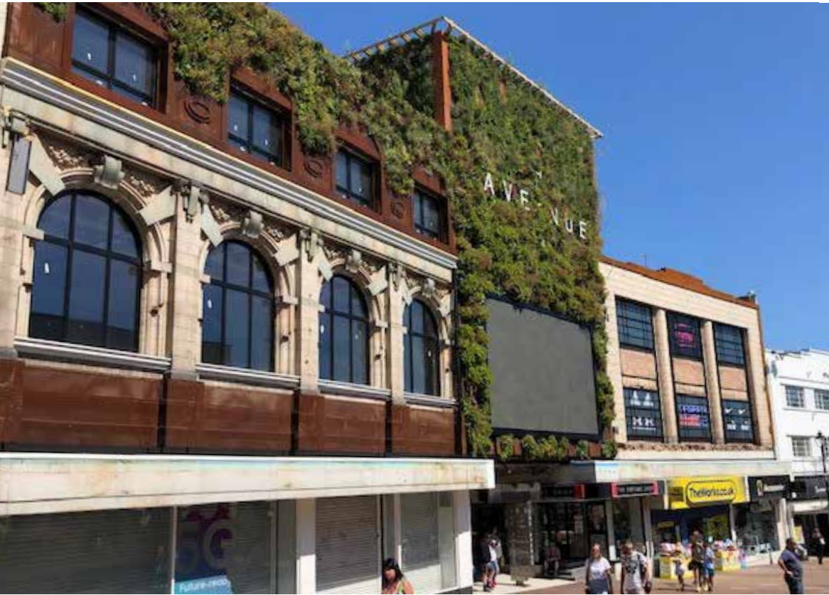
Commercial Road facade.
