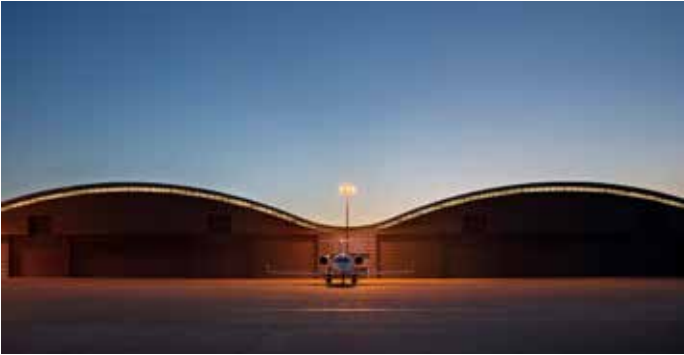
Industry & Technology / Farnborough Airport Hangars.
