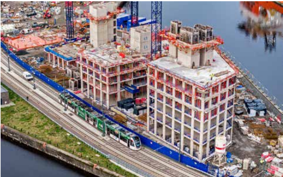
Currently under construction (2024).
