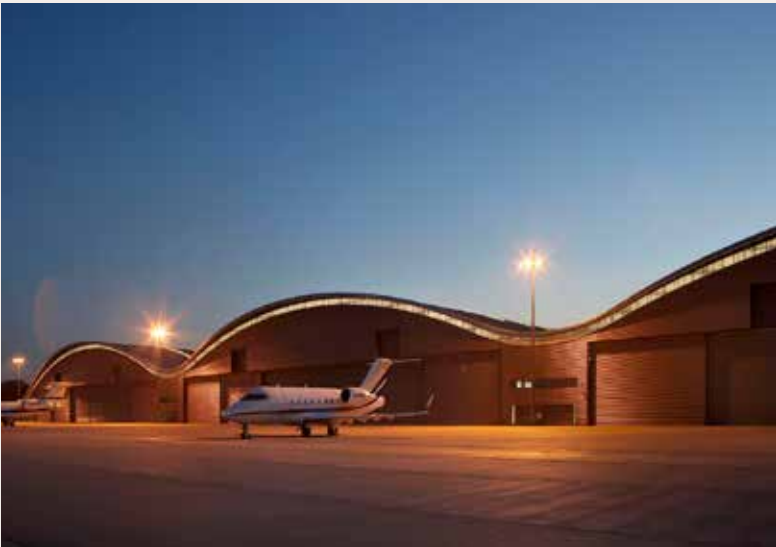
Farnborough Airport Hangars.
