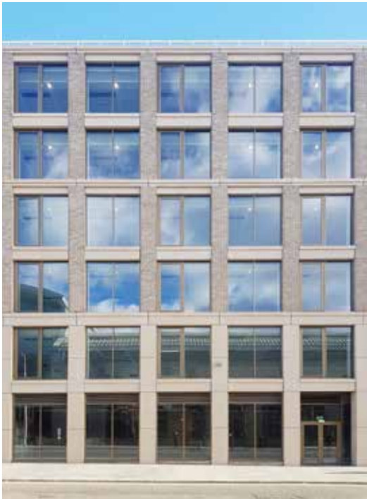
No2 Freer Street office facade.
