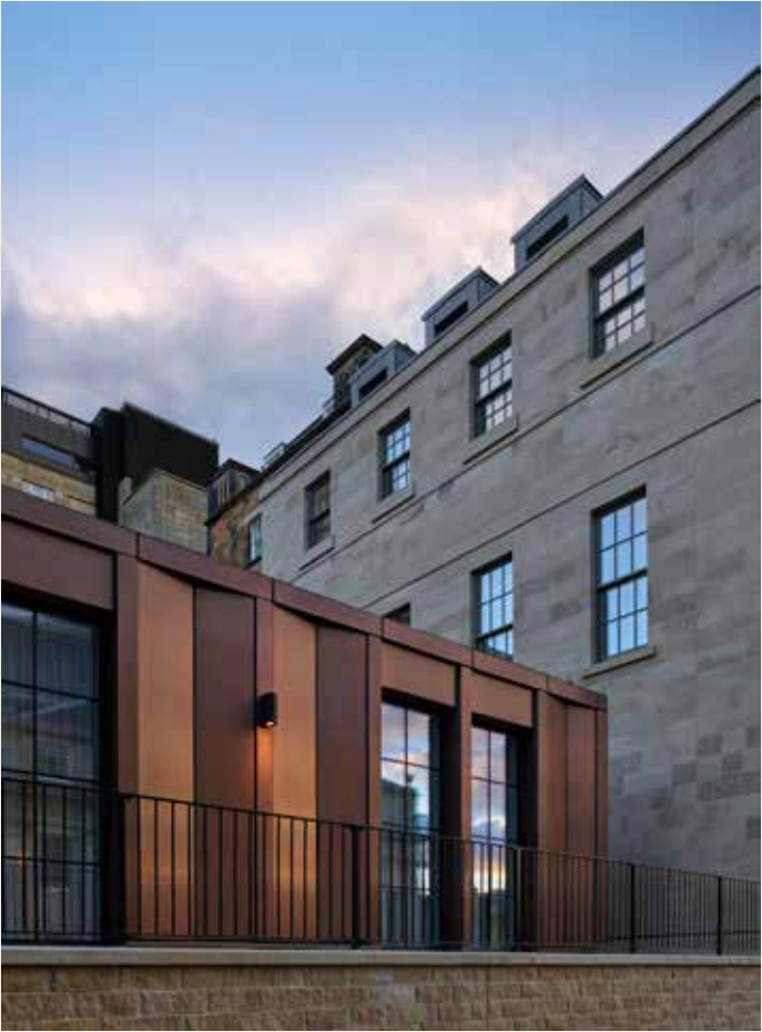
Townhouse extension and copper clad pavilion.
