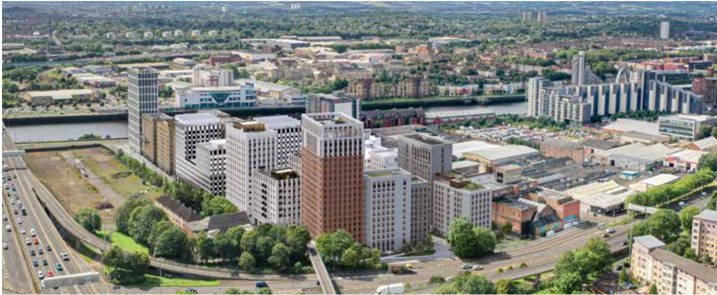
Aerial visual looking south.
