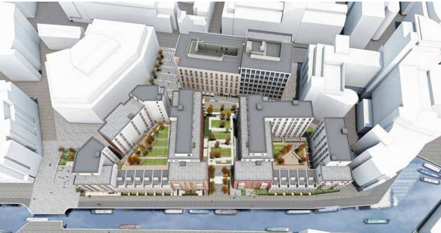
Aerial view from the southern edge.
