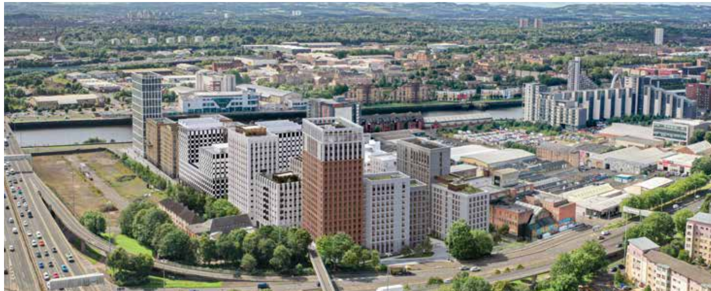
Aerial visual looking south.
