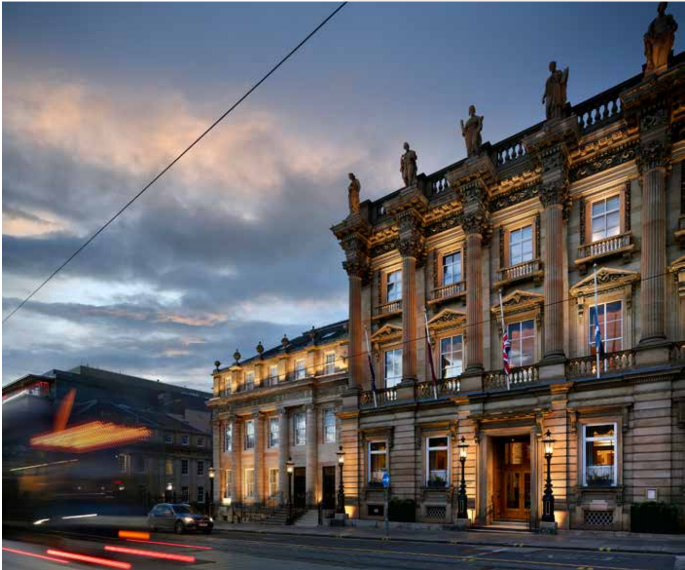
No. 39 St Andrew Square entrance.
