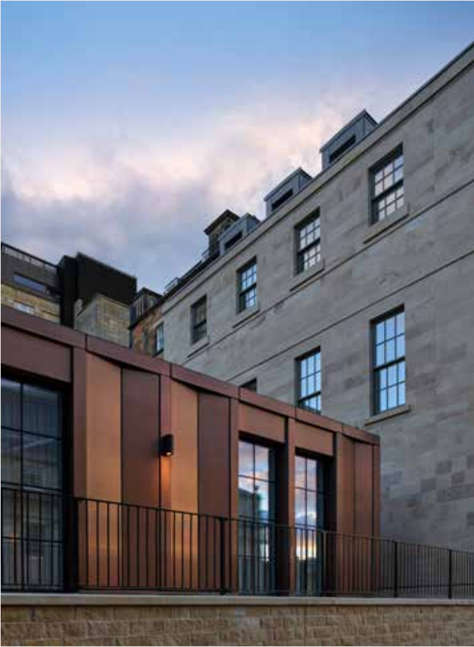
Townhouse extension and copper clad pavilion.
