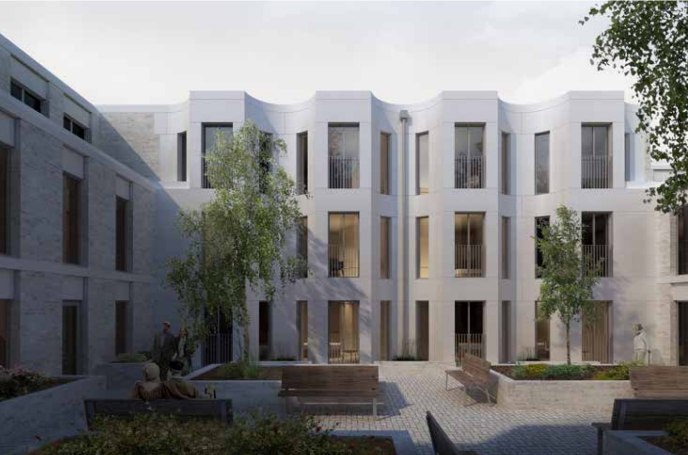
Dementia care accommodation: a domestic scale.
