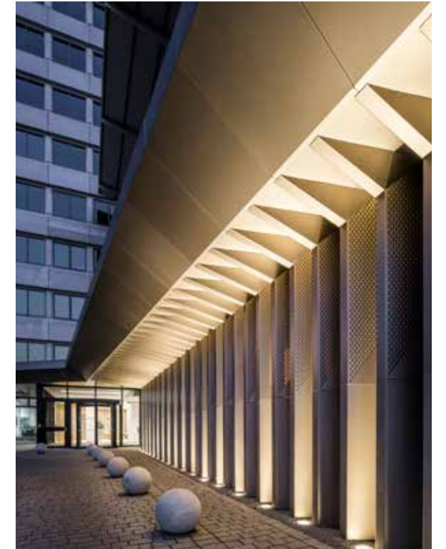
The Switch entrance.
