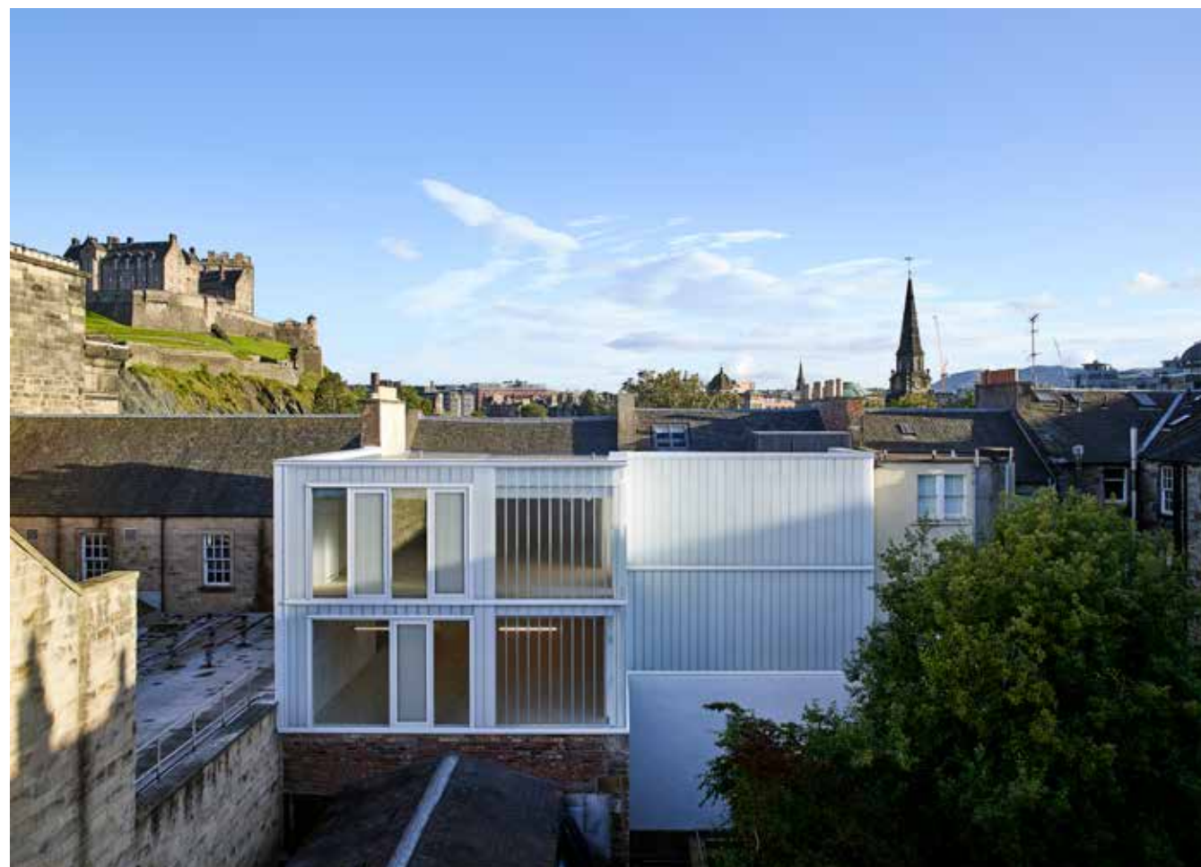
Contemporary extension to the rear of the building.
