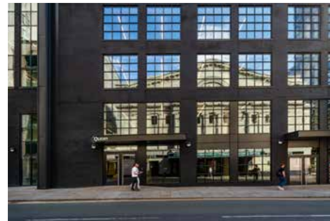
Quay Street facade.
