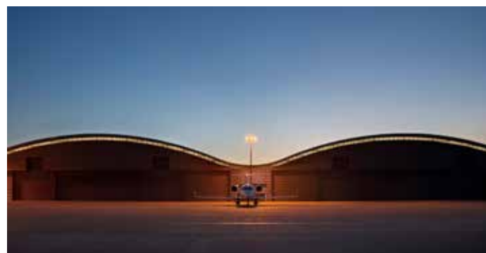
Industry & Technology / Farnborough Airport Hangars.
