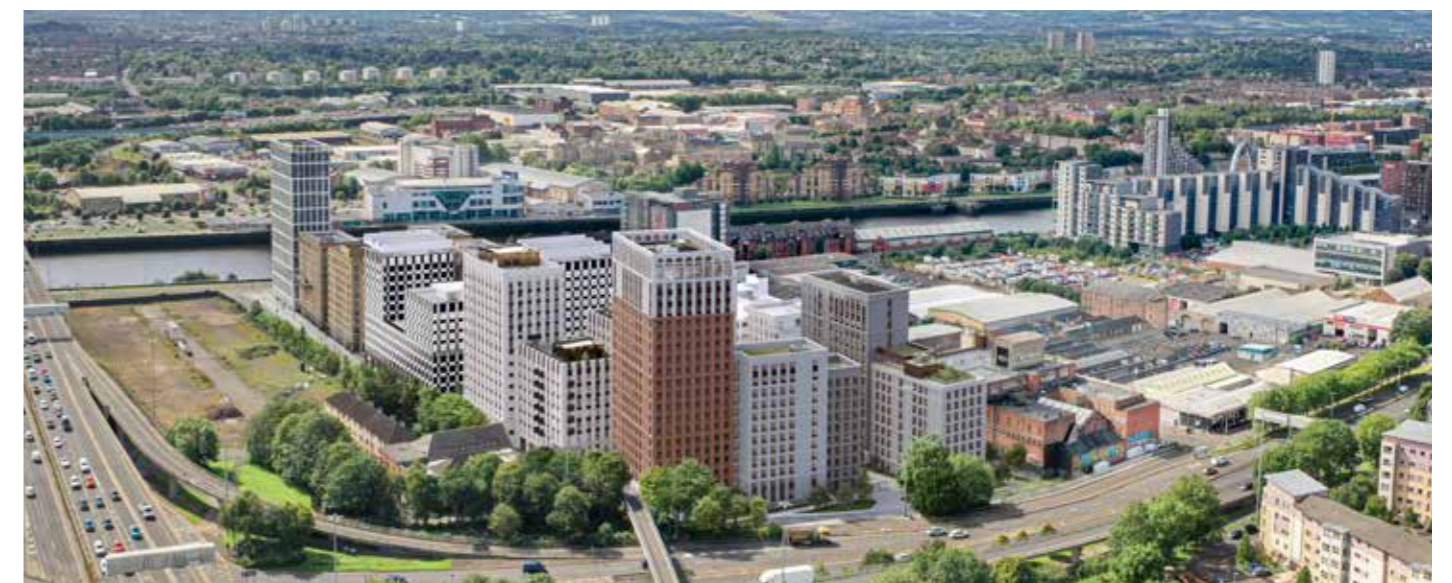
Aerial visual looking south.
