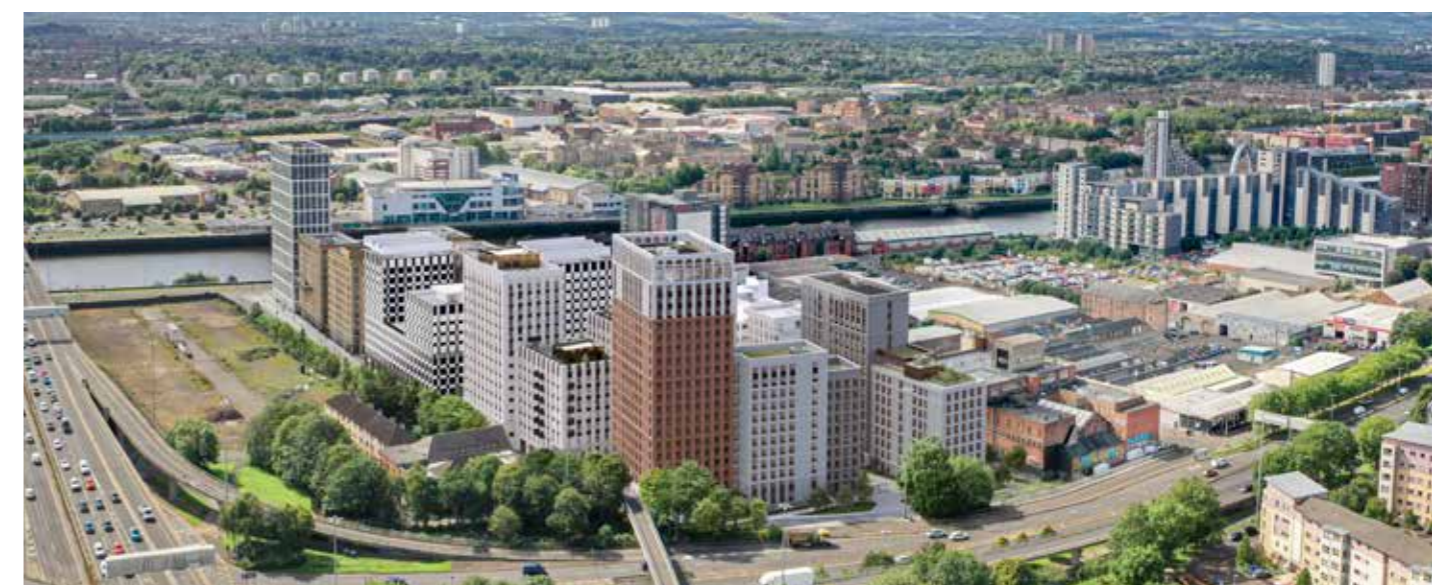
Aerial visual looking south.
