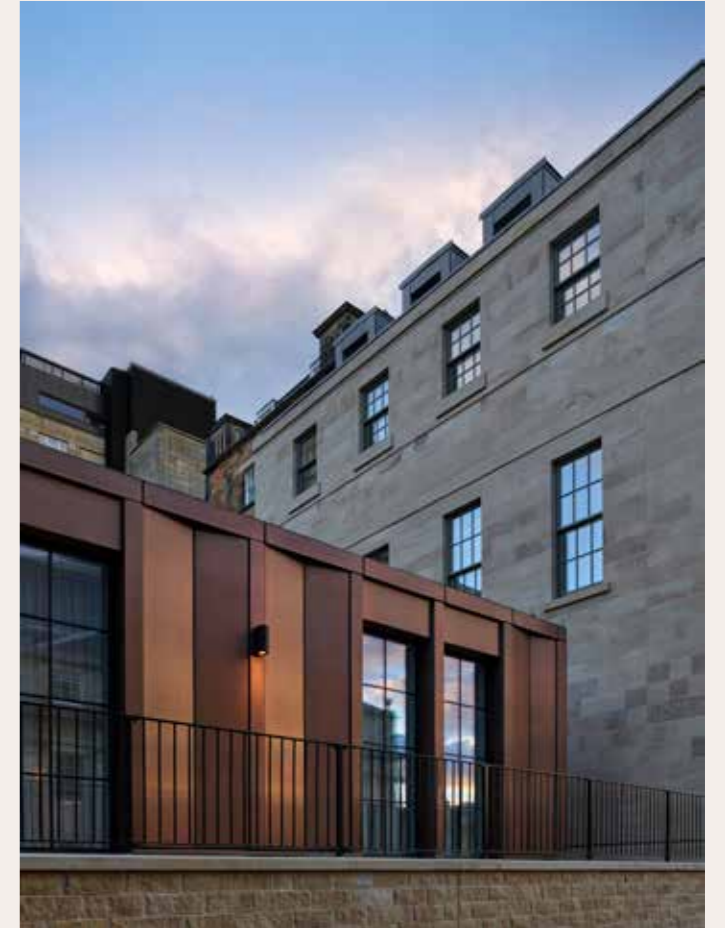
Townhouse extension and copper clad pavilion.
