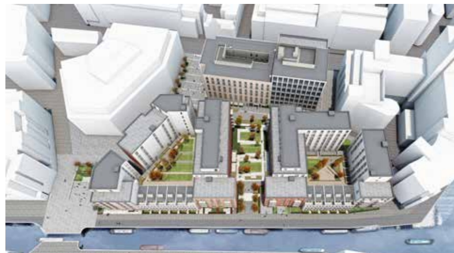
Aerial view from the southern edge.
