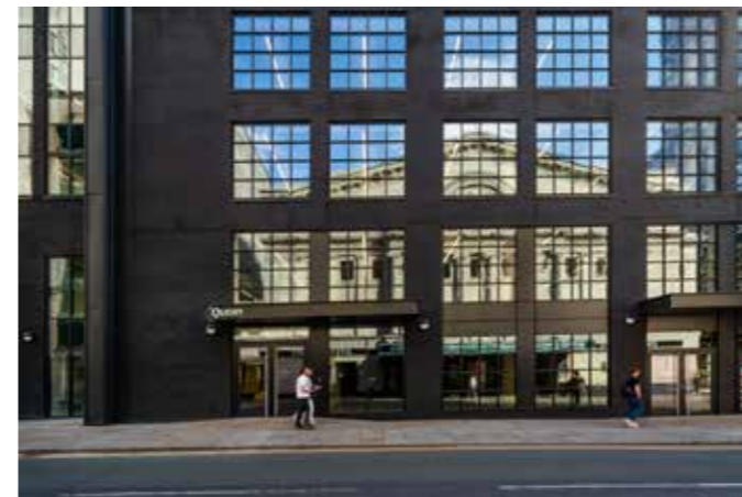
Quay Street facade.
