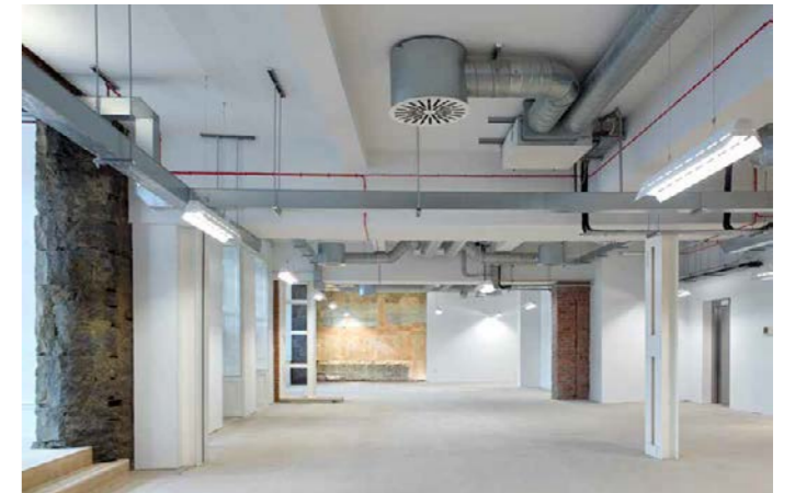
A key driver underpinning the scheme is to expose and enhance the historic fabric of the existing building to create character speculative office floorplates.
