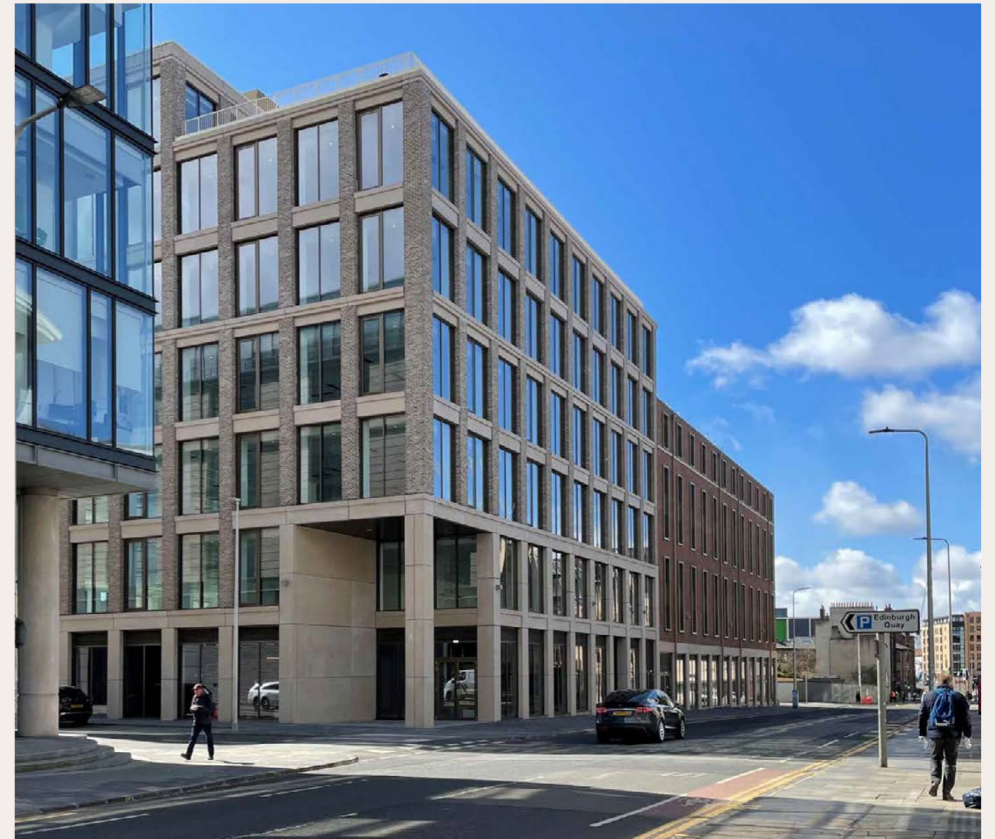
No2 Freer Street flexible Cat A office space.
