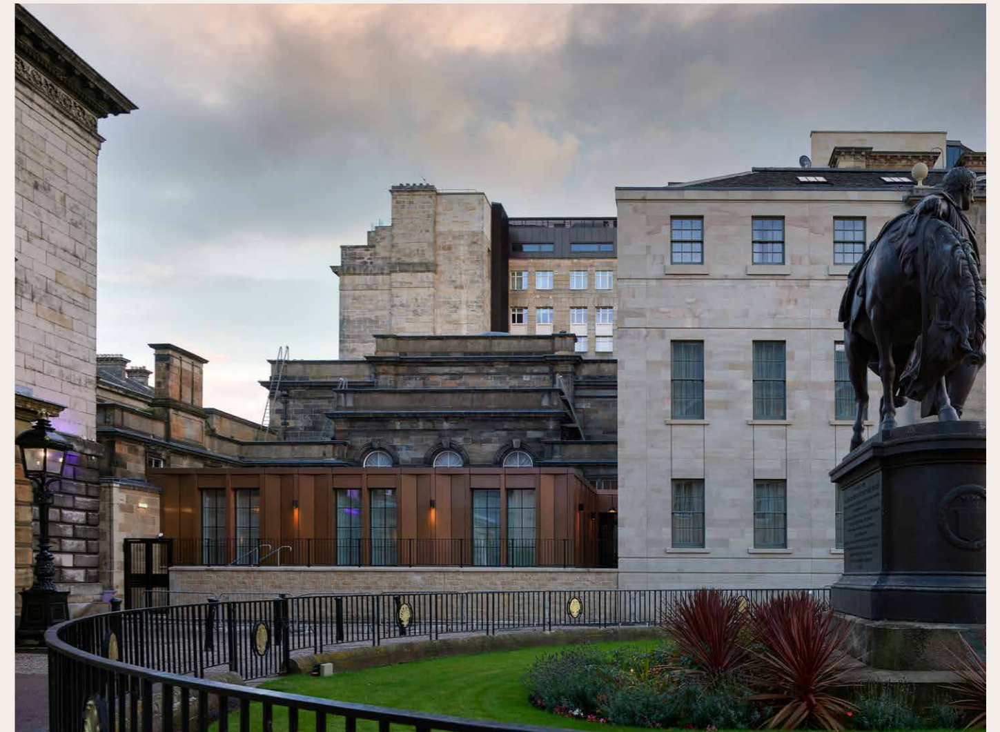
The Gleneagles Townhouse project both renews an existing building and extends it with a copper-clad 'pavilion' structure and a new masonry façade complementary to the setting.
