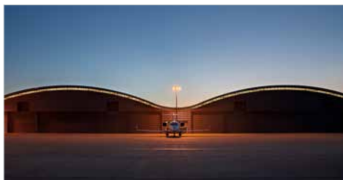
Industrial / Farnborough Airport Hangars.
