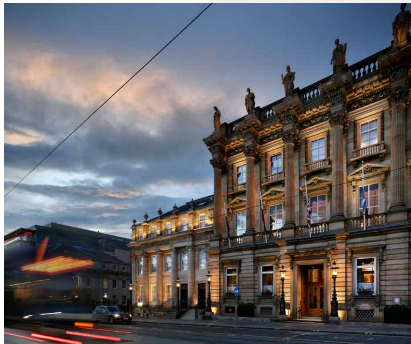
No. 39 St Andrew Square entrance.
