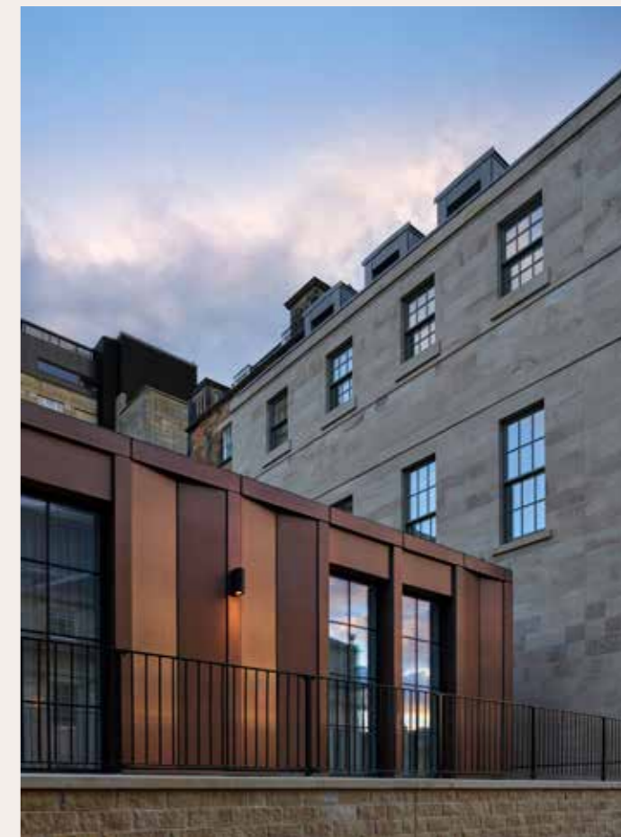
Townhouse extension and copper clad pavilion.
